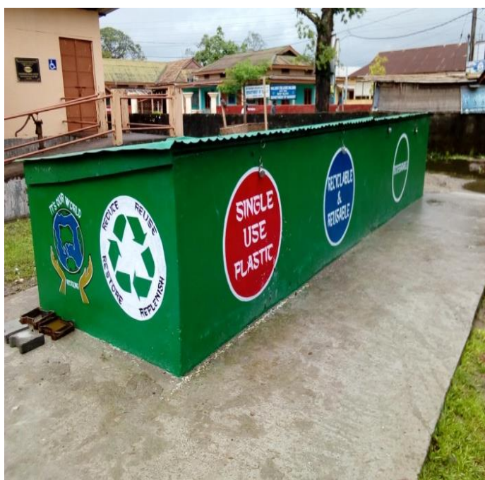
Cemented waste bin for the segregation of organic, inorganic and plastic waste.
