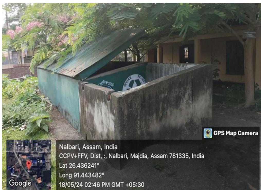
Cemented waste bin for the segregation of organic, inorganic and plastic waste.
