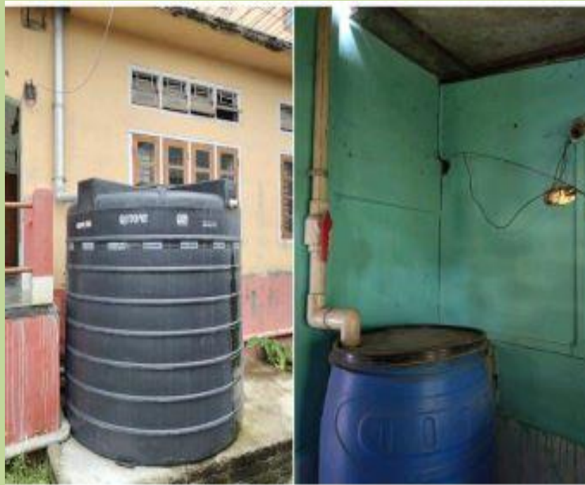
Rainwater harvesting facility at Nalbari College for water conservation: a scientific approach to water management
